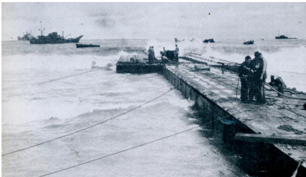
Figure 2-22 Resupply causeway, constructed by the US Navy's Seabees at Unai Chulu. (Hoffman 1951)
